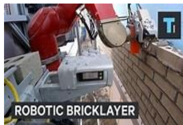
Fig 4.1 Robotic brick layer
